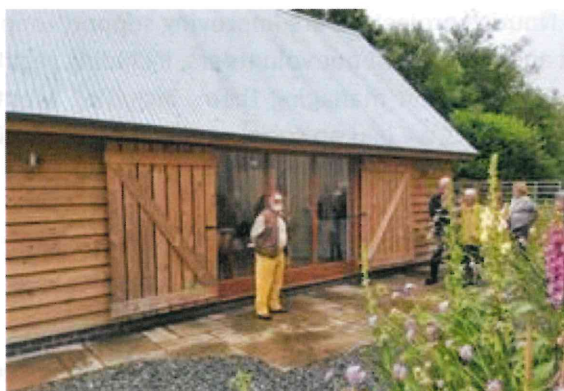
Formal opening of the Barn
