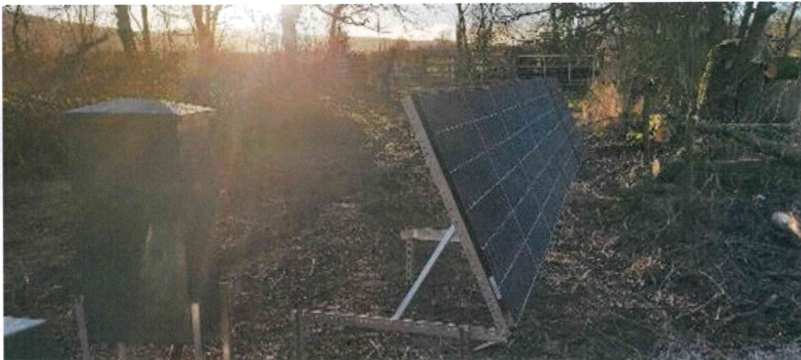
We installed a borehole and solar powered pump to provide water for cattle at Parky Meadow.
