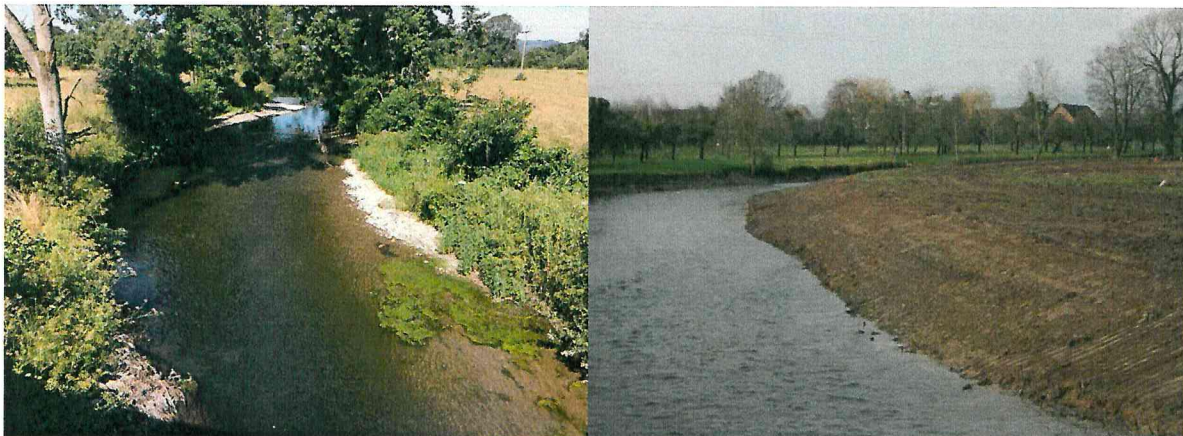
River Lugg, before and after the works
